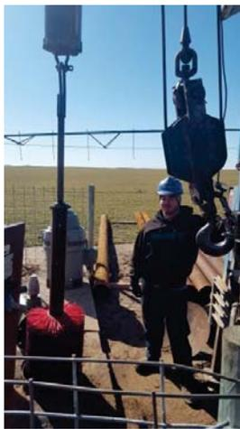
**Scrubbing-** Scrubbing is a weighted bristle-brush used to clean scale build up from the perforations. This tool is lowered down the hole and worked vigorously up and down creating a wire brushing effect. When coupled with a video and other rehabilitation methods, scrubbing can become a precise and an effective means to increase flow.
